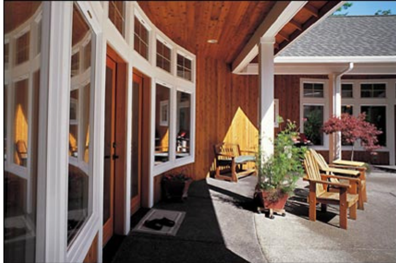
The sweep of the wall connects two separate living suites at the courtyard. Columns help bear the weight of the roof, taking the stress off the wall, so the curve does not have to align with its support.
